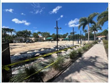
The Tennis Court 5-7 HydroCourt Project is in its second week and well ahead of schedule. All Hydration boxes are in place, all plastic liners are installed, all piping and hydration mats are installed. Screening material (sand) has been installed on all of the courts. After hydrating and rolling the screening material, Ritzman will begin adding the Har-Tru clay, this may happen as early as next week.
